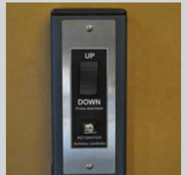
Key Switched Controls
