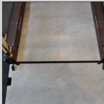
Special Floor Covering
