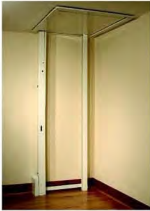
Lower room when lift upstairs
